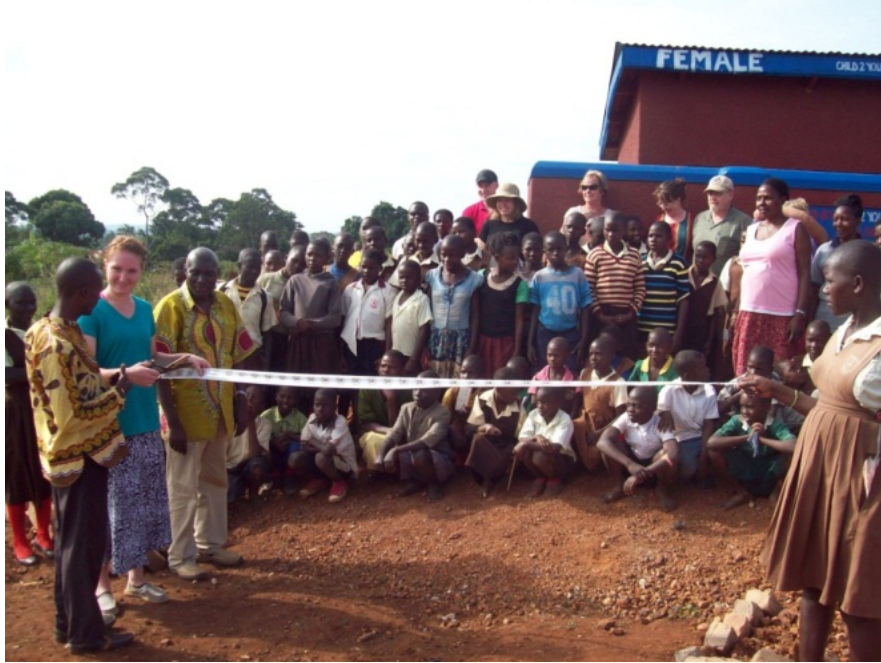
The completed lined pit latrine being handed over to the school. The ceremony was done and witnessed by US visitors from Idaho, one of the visitors is preparing to cut the tape while Steven, Headmaster of the school and school children are looking on.
